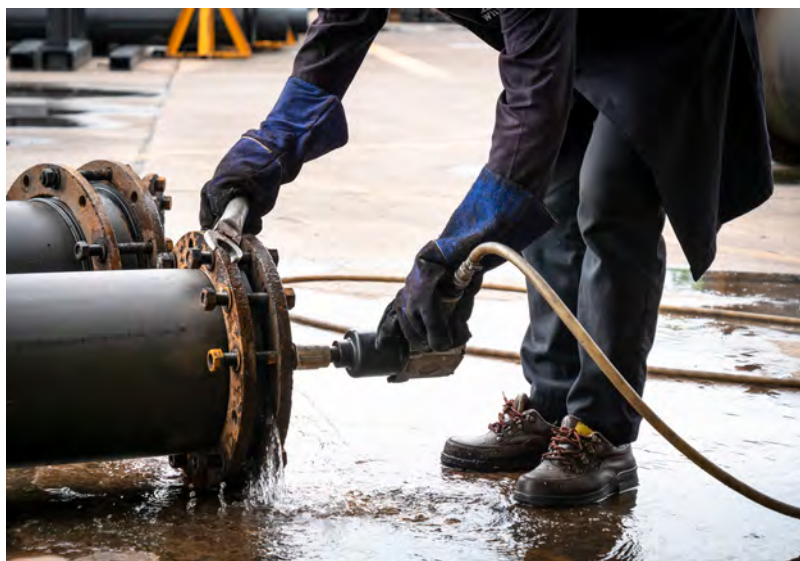
Figure 1. Performing a pipeline hydro test.
