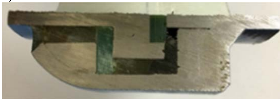
Figure 6: Void between pipe and collar
