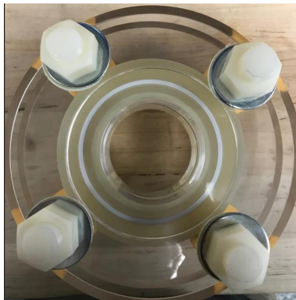
Image 3: A look down the flange bore with a properly sized gasket
